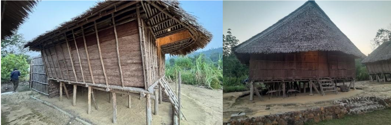
Figure 5. Memarong Unjem piles (left) and Memarong Lantok piles (right)
