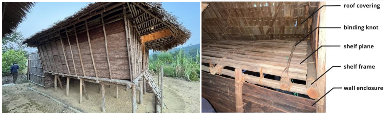
Figure 7. Memarong wall's side view (left) and the wall shelf inside (right)
