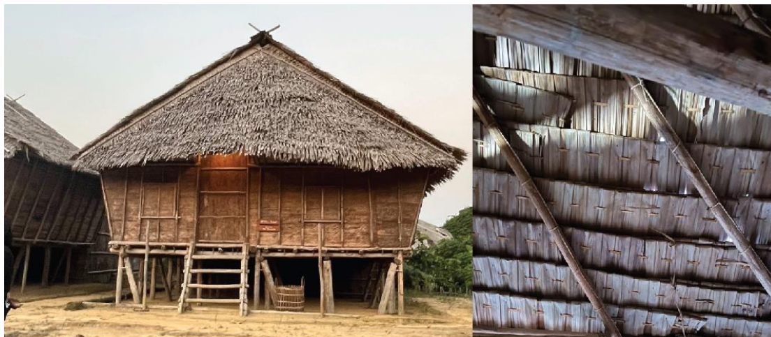
Figure 6. Memarong roof profile (left) and the roof details (right)
